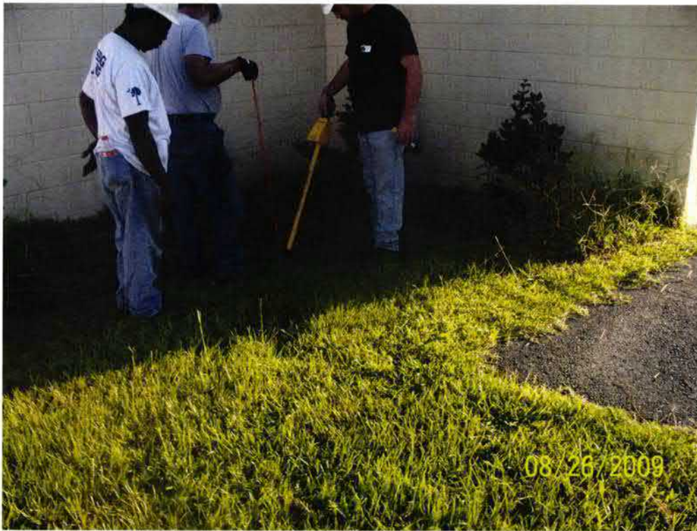
Picture 1: Location of UST 1231Dove.
