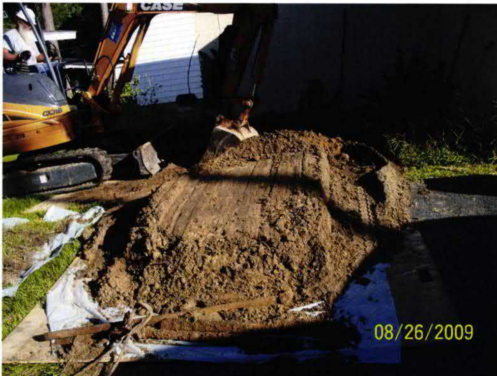
Picture 2: UST 1231Dove removal in progress.
